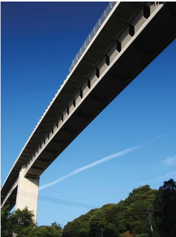
FIGURE 1 View of the Takubogawa Bridge
